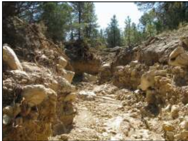
What had been a minor drainage was ripped by water to expose huge boulders and tear ponderosas that were carried to the river below.
