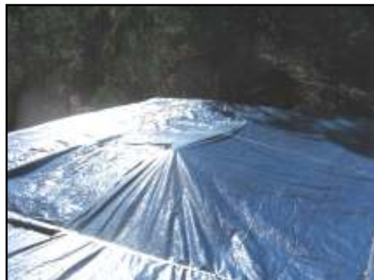
Roof tarp in place; center bulge is roof entry
